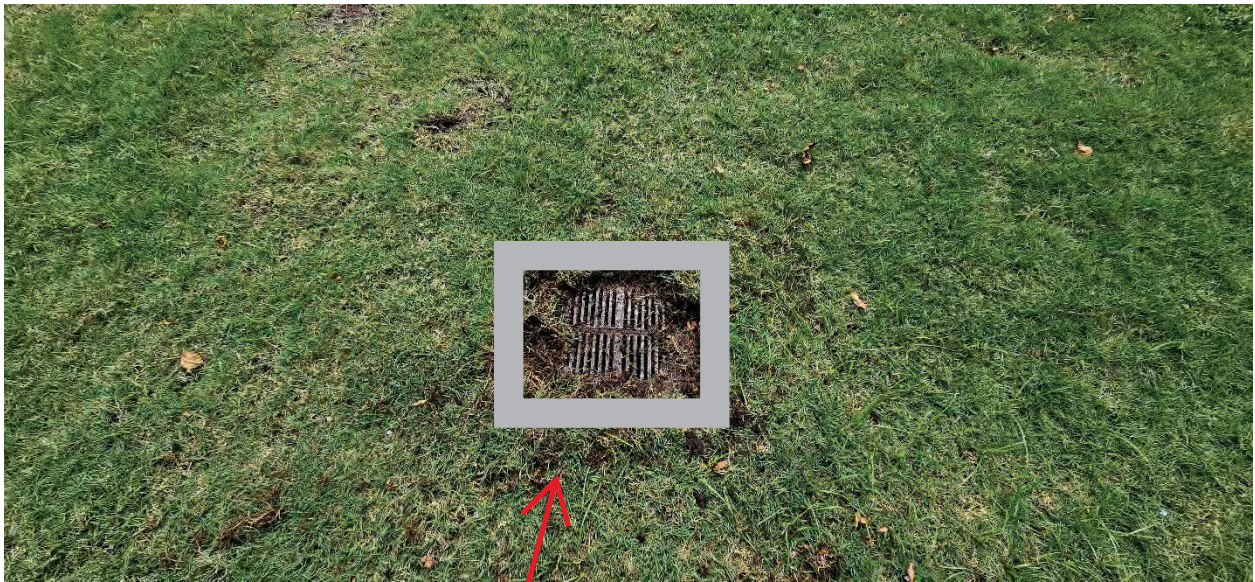
8" Concrete ribbon around drain.
